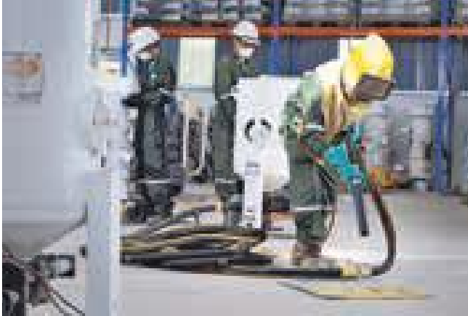
Blasting using Sponge Jet Technology
