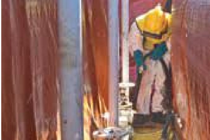
Blasting using Sponge Jet technology
