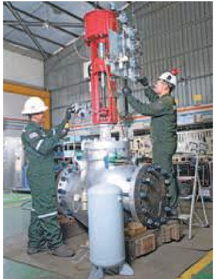
Calibrating and setting of turbine bypass pressure control valve
